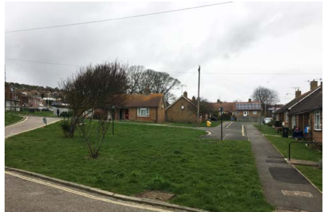
Bungalows at the northern end of the site.
