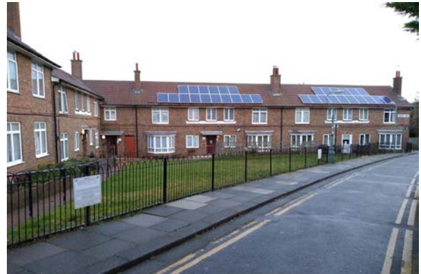
The building zig-zags across the site with anonymous triangular lawns to the front
