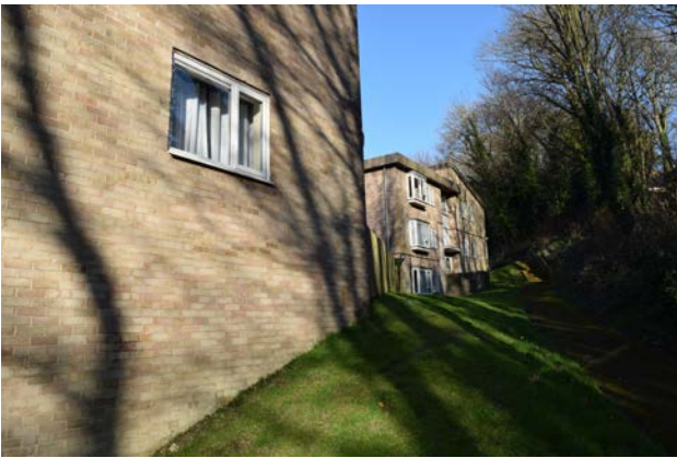
The sloping creates void areas below accommodation.
