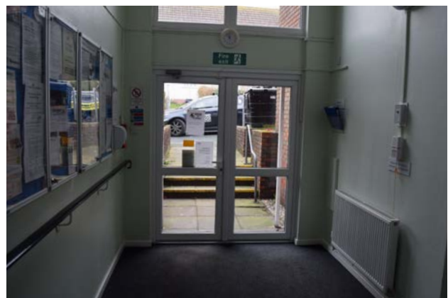
The secondary entrance does not provide level access, electric doors or a draught lobby
