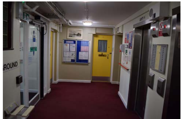
The entrance lobby is undersized and highly cluttered with exposed services and signage
