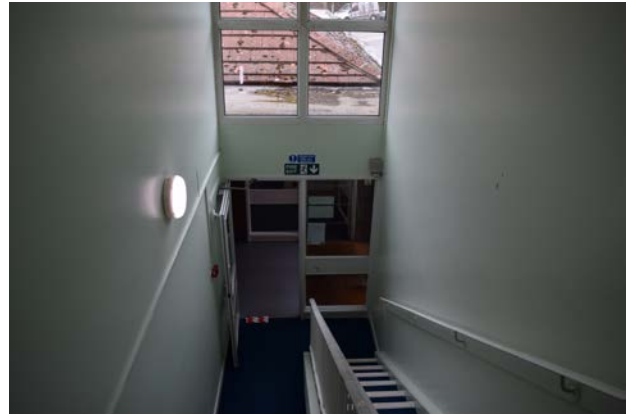
Circulation spaces are not designed to be wheelchair accessible
