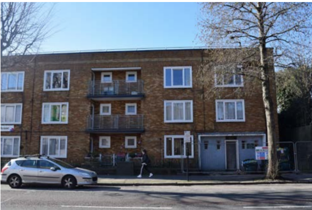
Former public toilets are being converted into a communal lounge
