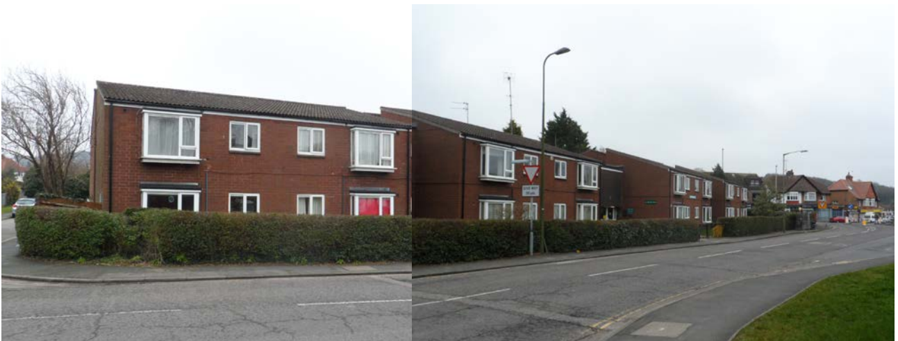
Panoramic view of the front of Jasmine Court. The building is formed of low-rise individual blocks linked together on a busy road.
